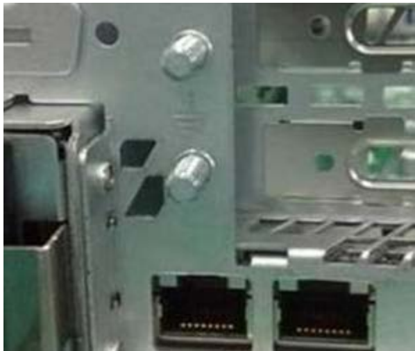
Figure 1: The ground studs
