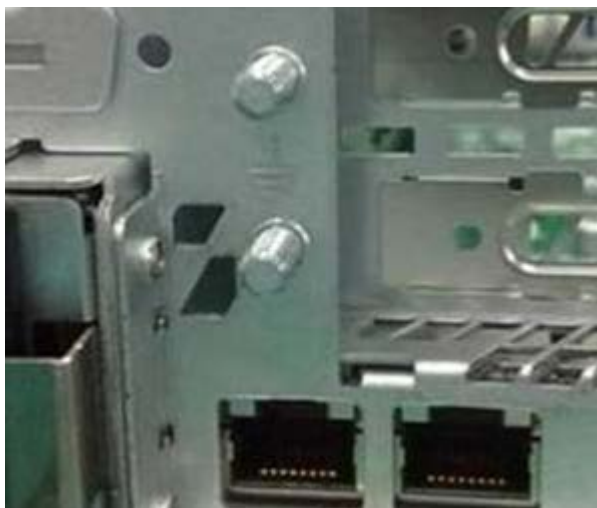
Figure 1: The ground studs
