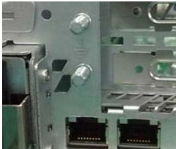
Figure 1: The ground studs
