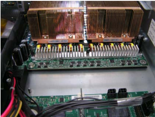
Old 80mm fans mounting location (Note: fan module is removed)
